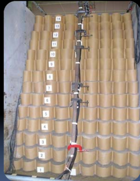
Cheaper way to stabilize slope
