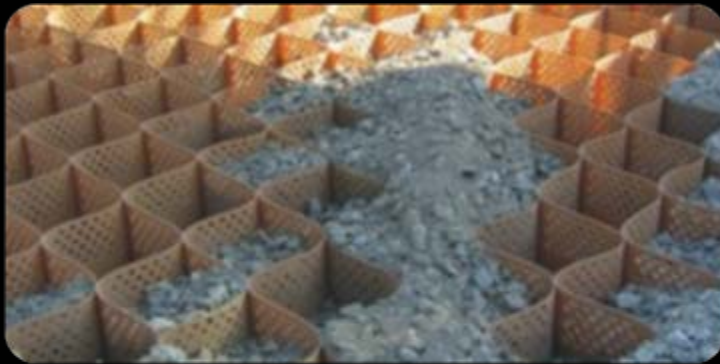
Roadbed test section
